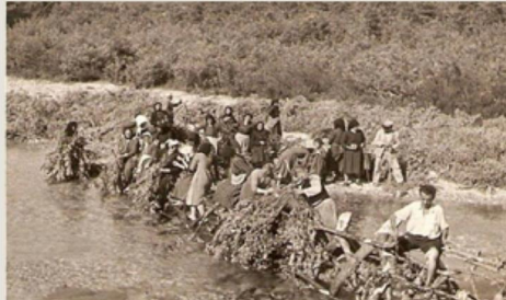
Construction of an artificial dam in the river to divert water towards the fields
